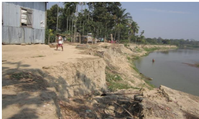
Fig 7: The vulnerable position of the houses along the Khowai River at Purba Kalyanpur.
