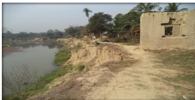
Fig 5: The vulnerable position of the houses along the Khowai River at Moharchhara
